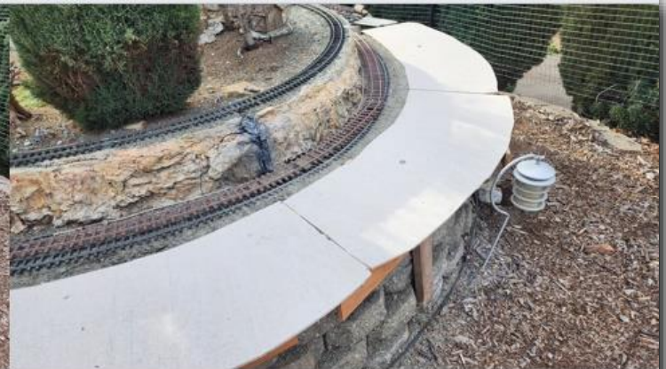
Enlarged cement board platform from installed.
